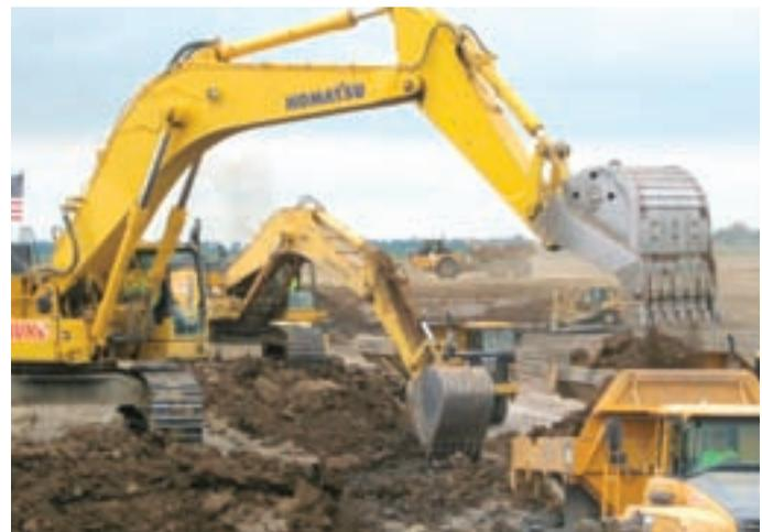
**To track production on the site, Nick Savko & Sons installed Trimble CrossCheck devices on almost every piece of equipment and reviewed reports in real time in Trimble Construction Manager software.**
